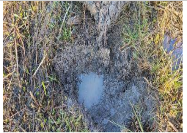
IMAGE 2 LOW-LYING WET AREA TEST PIT IN PROGRESS
