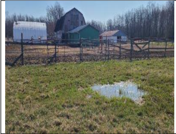
IMAGE 13 LOW-LYING WET AREA AND BARN COMPLEX
