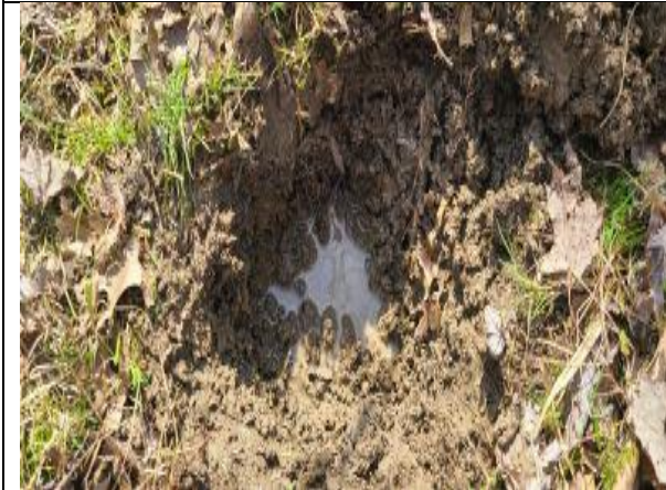
IMAGE 11 LOW-LYING WET AREA TEST PIT IN PROGRESS
