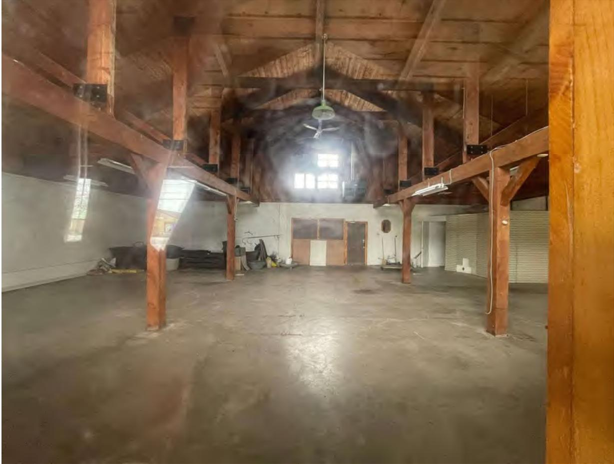
Photograph No. 6 – Interior of the commercial building. Concrete poured floors, wooden trusses, and drywall were utilized for the interior building materials.
