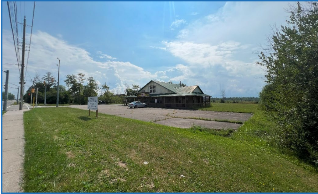
Photo 1 – View from northwest corner of the Subject Lands looking southeast, with existing vacant structure shown (centre) to be demolished as part of proposal.
