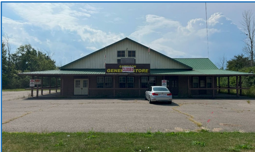
Photo 2 – View of existing vacant structure to be demolished, looking south from Garrison Road.
