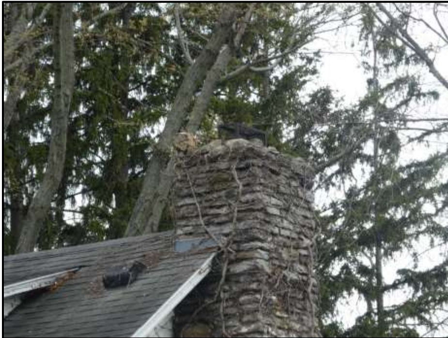
Photograph 15. Residence Chimney with Wildlife Exclusion Covering
