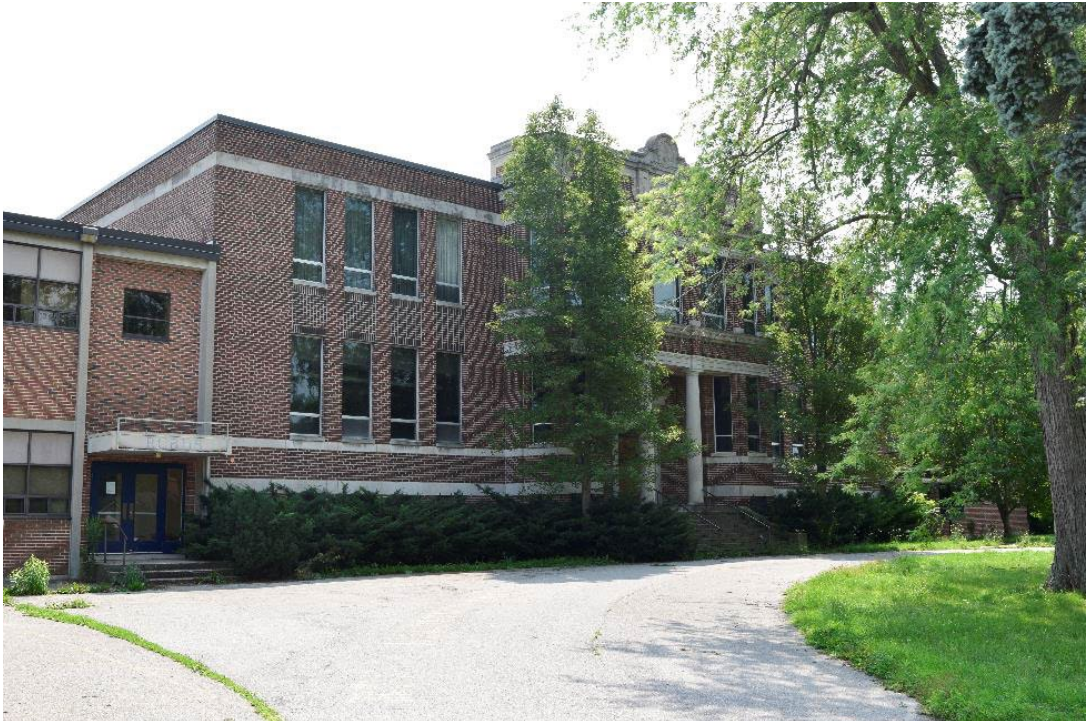
Image 2: Northwest corner of structure
