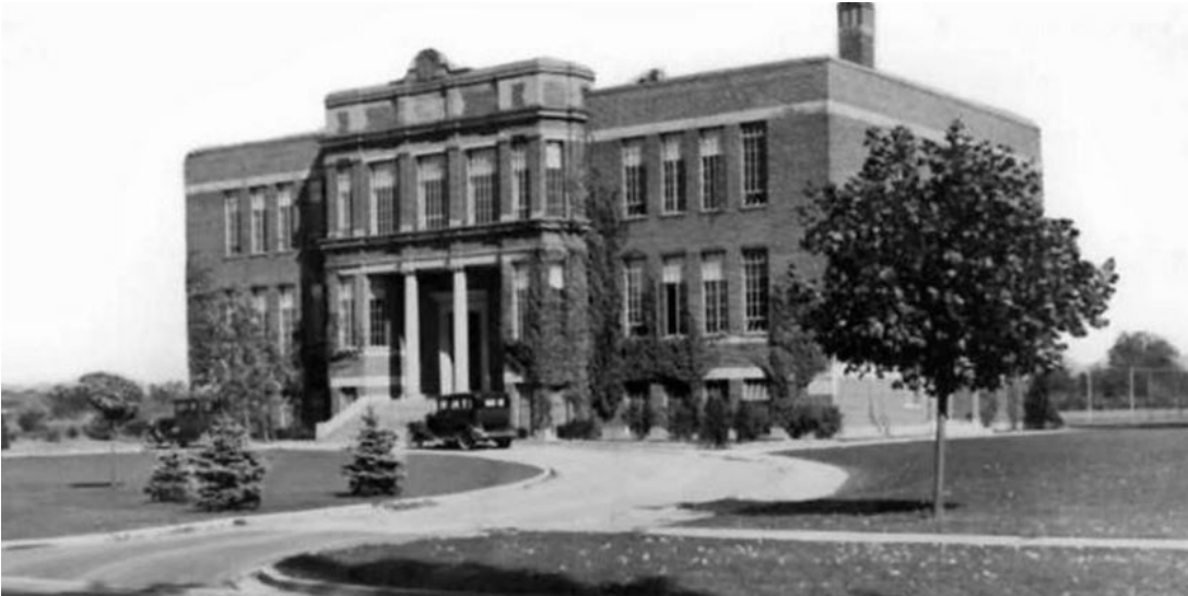
Image 9: Undated photo of original structure
