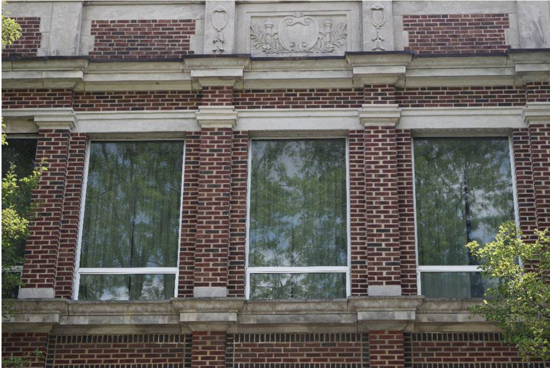
Image 7: Typical replacement windows in 1927 structure
