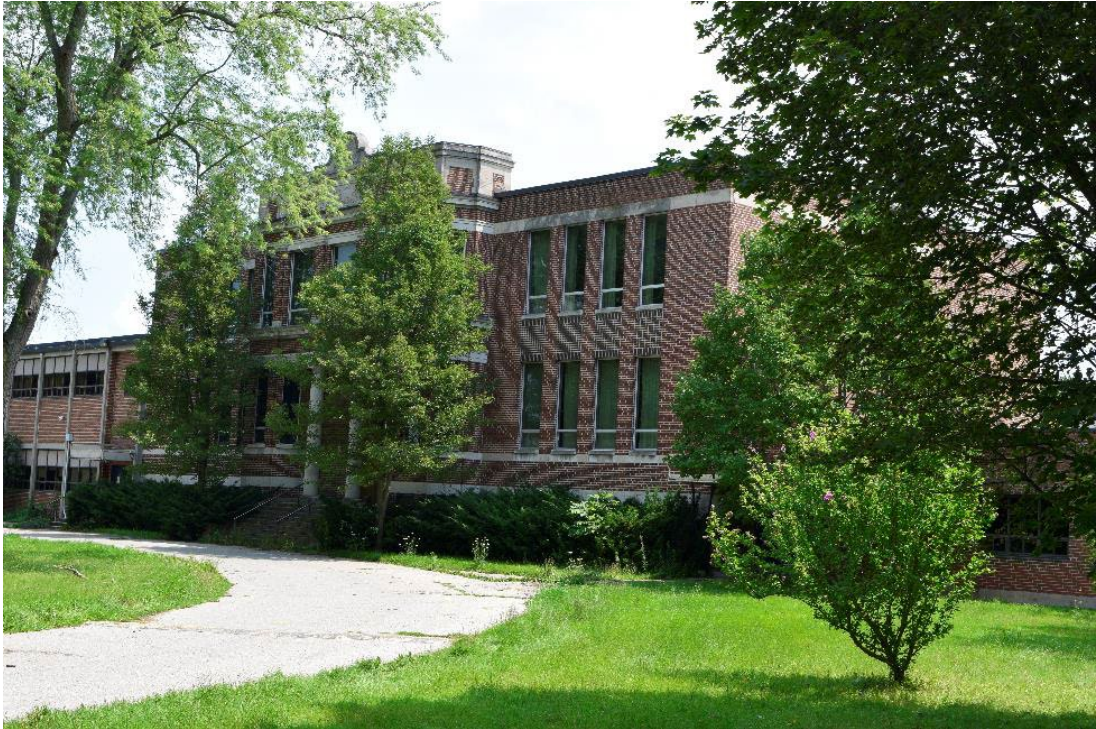
Image 3: Southwest corner of structure
