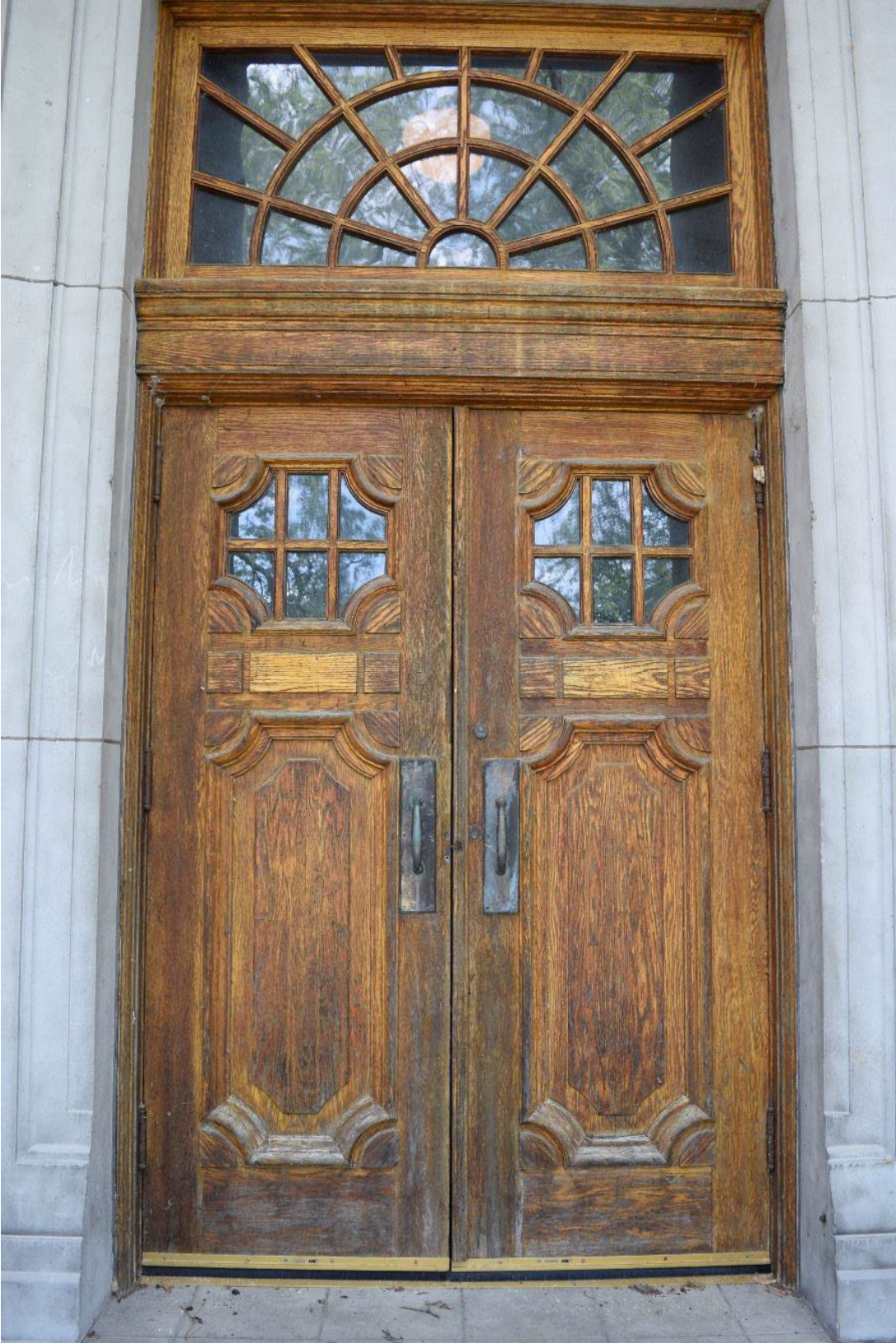
Image 4: Original wood front doors and transom of front entrance
