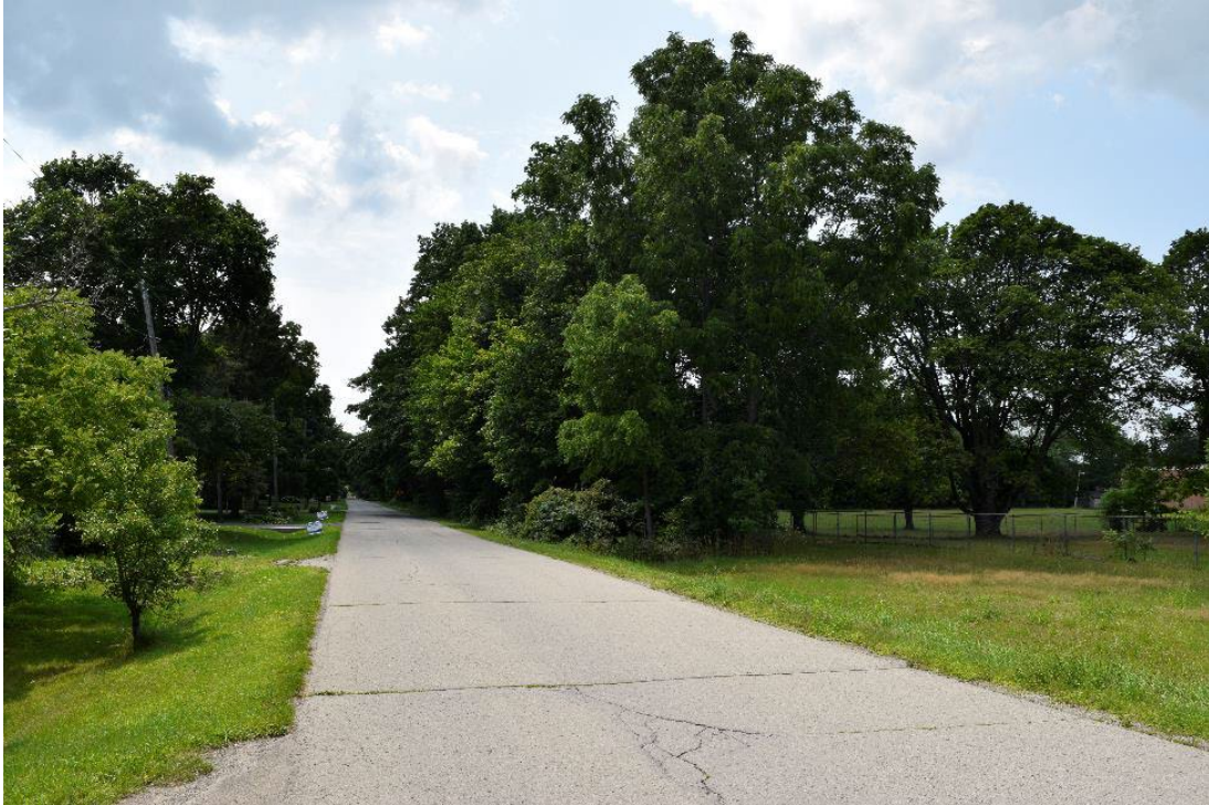
Image 16: Typical tree cover indicative of southeast exposure to Prospect Point Road North
