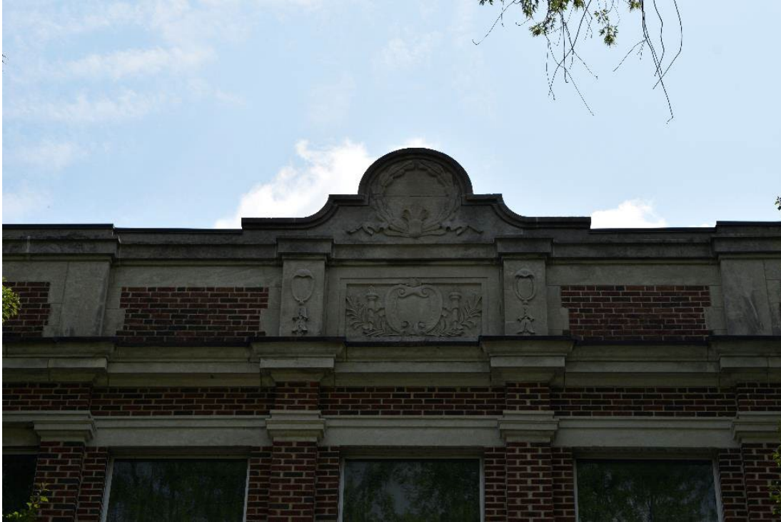
Image 6: Details on parapet over front entrance
