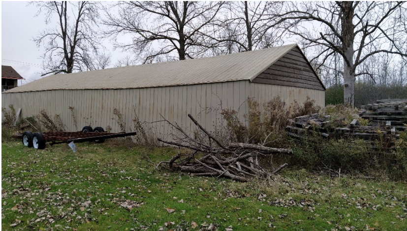
View of the southwest elevation of the storage structure on the Subject Property, looking northeast.
