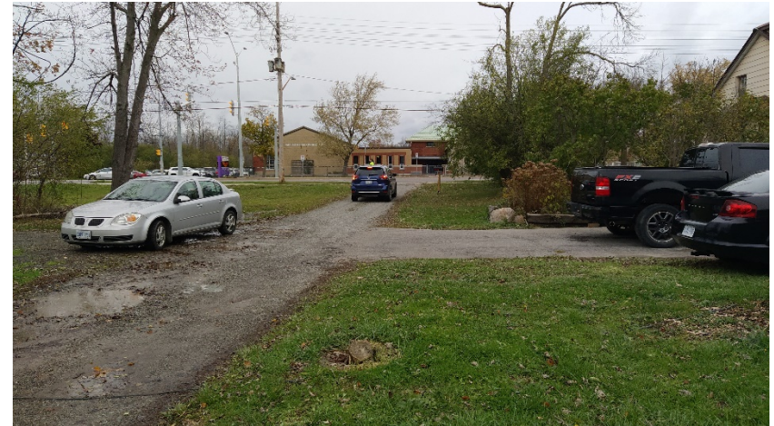
View of the asphalt paved and gravel covered driveways on the west portion of the Subject Property, looking north.
