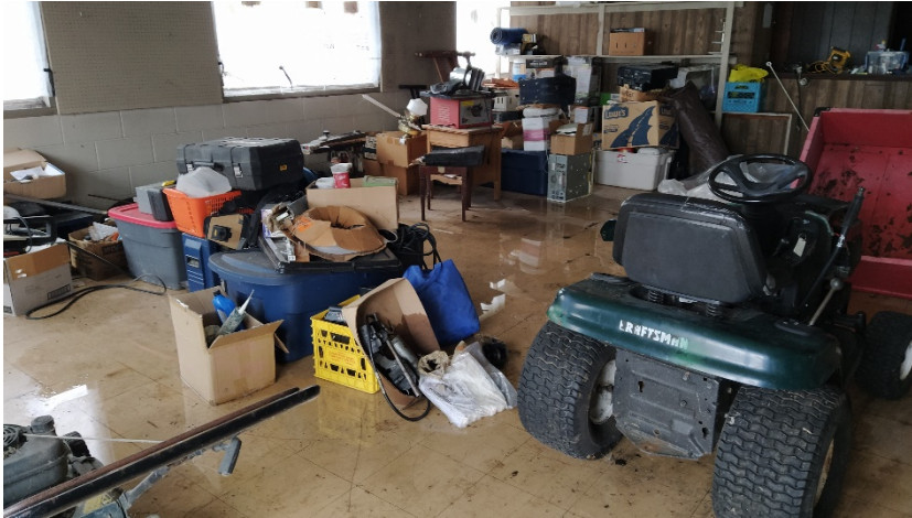
View of the vinyl floor tiles within first floor garage area of Site Building 2.
