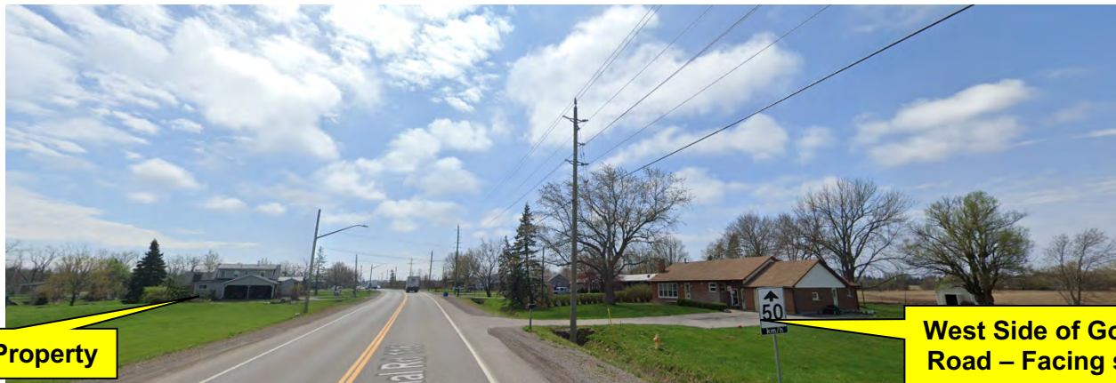
Figure 6 – Across the Street, Opposing Side of Gorham Road (West) (Google Maps, 2021)
