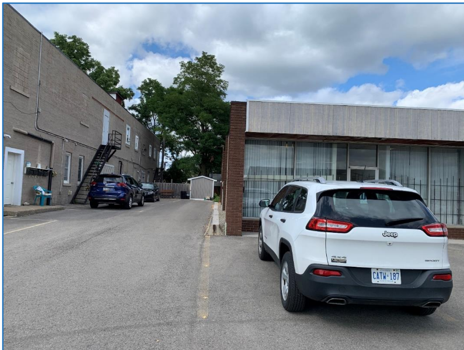
Figure 4. View looking north on Courtwright Street towards the commercial structure to the east of the Subject Lands (Subject Lands are on the left)
