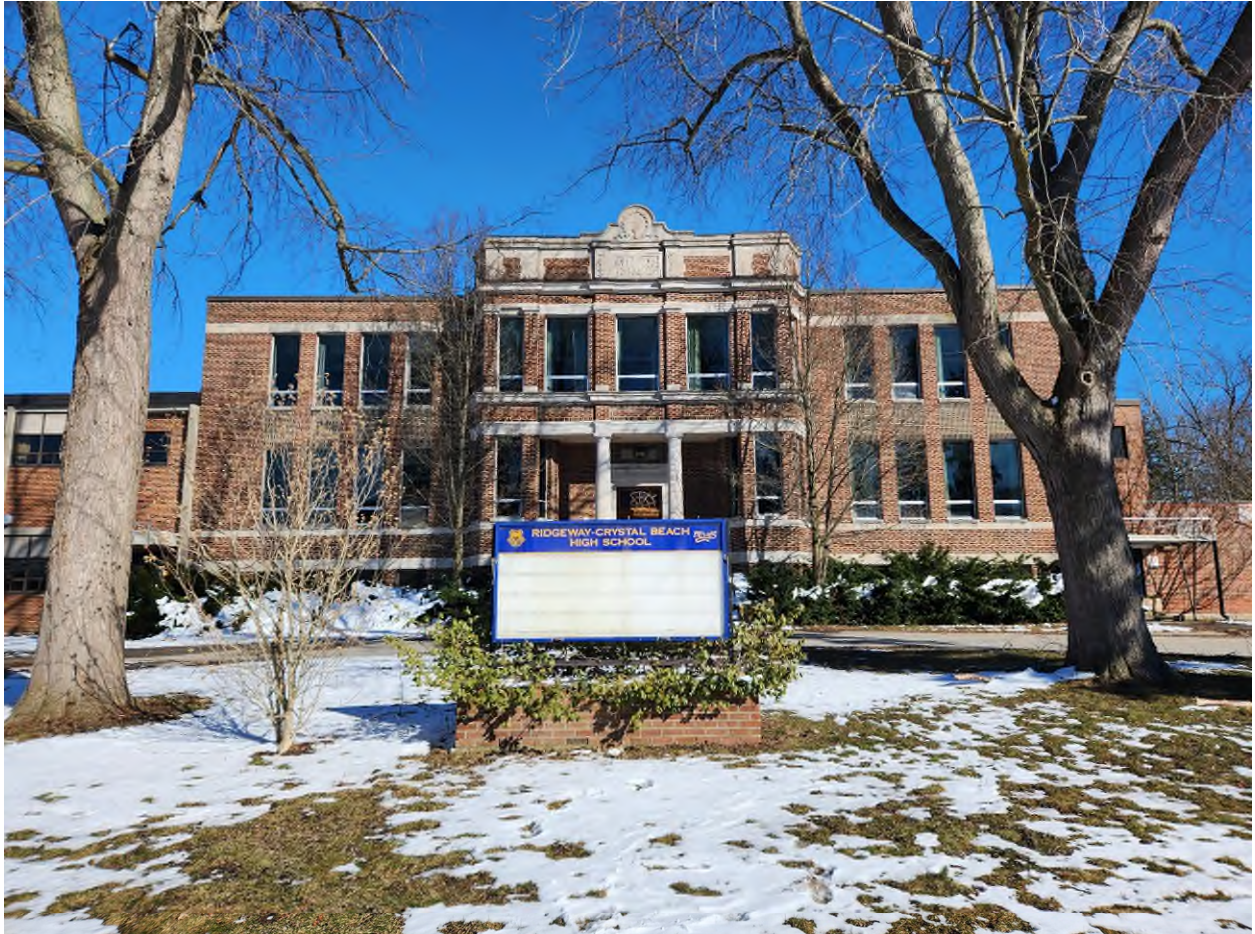
Figure 3 - Original Building Facade
