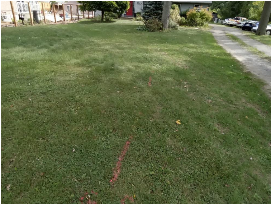
Image 6: View of portion of the front yard showing marked buried utility locates between road and house.
