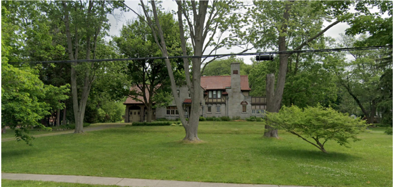
Figure 8 – Existing Heritage-designated Dwelling at 546 Ridge Road North
