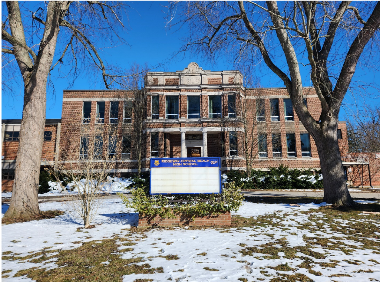
Figure 2 - Front Facade of the Original School Building
