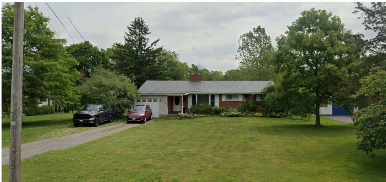
Figure 6 - Existing Dwelling at 630 Prospect Point Road
