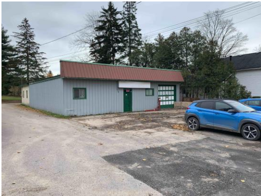
Photo 5: Existing building and paved driveway; facing east
