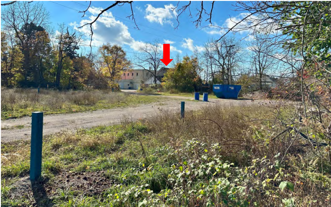
FIGURE 7: VIEW TOWARDS STRUCTURE LOCATED AT 402 RIDGE ROAD NORTH FROM PROPERTY LINE BETWEEN 402 RIDGE ROAD NORTH AND SUBJECT PROPERTY, VACANT LAND SHOWN IN IMAGE WILL NOT BE IMPACTED BY PROPOSED DEVELOPMENT, HERITAGE STRUCTURE AT 402 RIDGE ROAD NORTH ILLUSTRATED WITH RED ARROW
