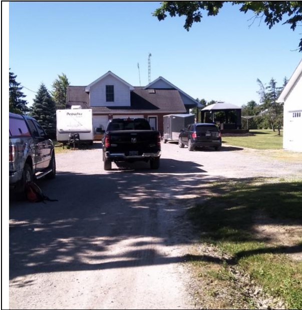
IMAGE 1 DRIVWAY AND STRUCTURES
