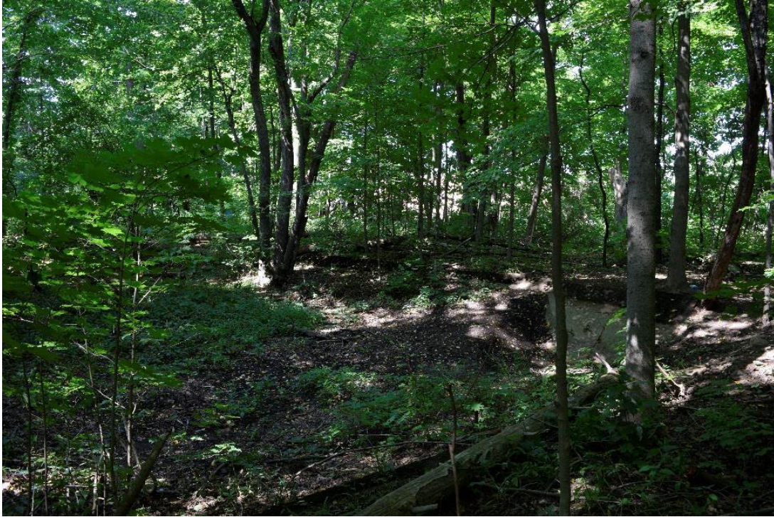
Figure 21: 25 m x15 m cement lined depression, looking northeast towards 576 Ridge Road North
